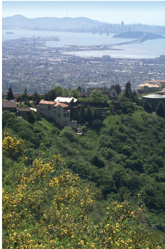
Hillside homes near wildlands are most at risk.
